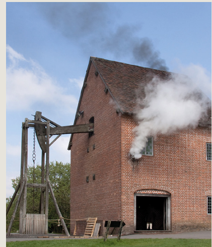
Image: A replica of Thomas Newcomen's 1712 steam engine, used to pump water out of tin and coal mines during the industrial revolution.
